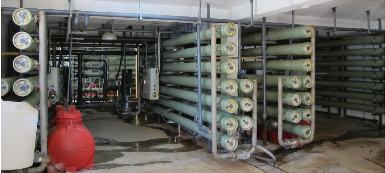
Figure 2: Brackish water RO-System for drinking water supply in Jerash, Jordan, operated by the Jordanian water authorities (photo: Oliver Jung)
