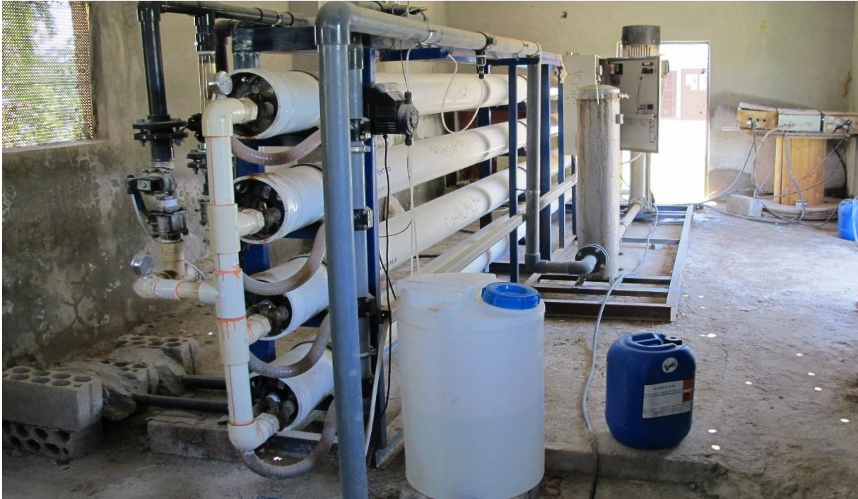
Figure 3: Typical RO-unit on a farm in Jordan (photo: Oliver Jung)
