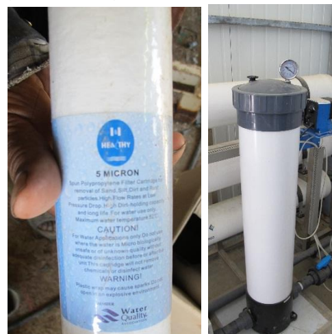
Figure 9: 5 \mu\text{m} filter cartridge and cartridge filter of a RO treatment plant in Jordan (photos: Oliver Jung)
