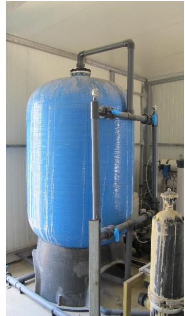
Figure 8: Sand filter of a RO treatment plant on a farm in Jordan (photo: Oliver Jung)
